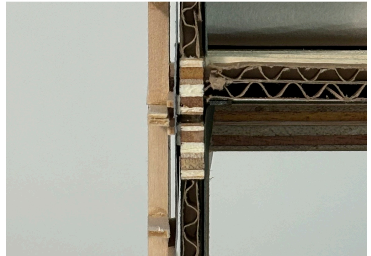
Close-up shots of the "chunk" model highlighting OSB and polycarbonate cladding connections, respectively.
