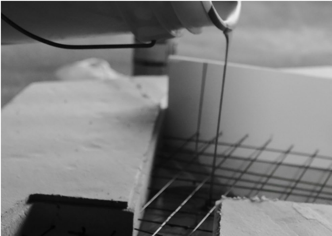
Process photos documenting the fabrication of the poured reinforced concrete base.
