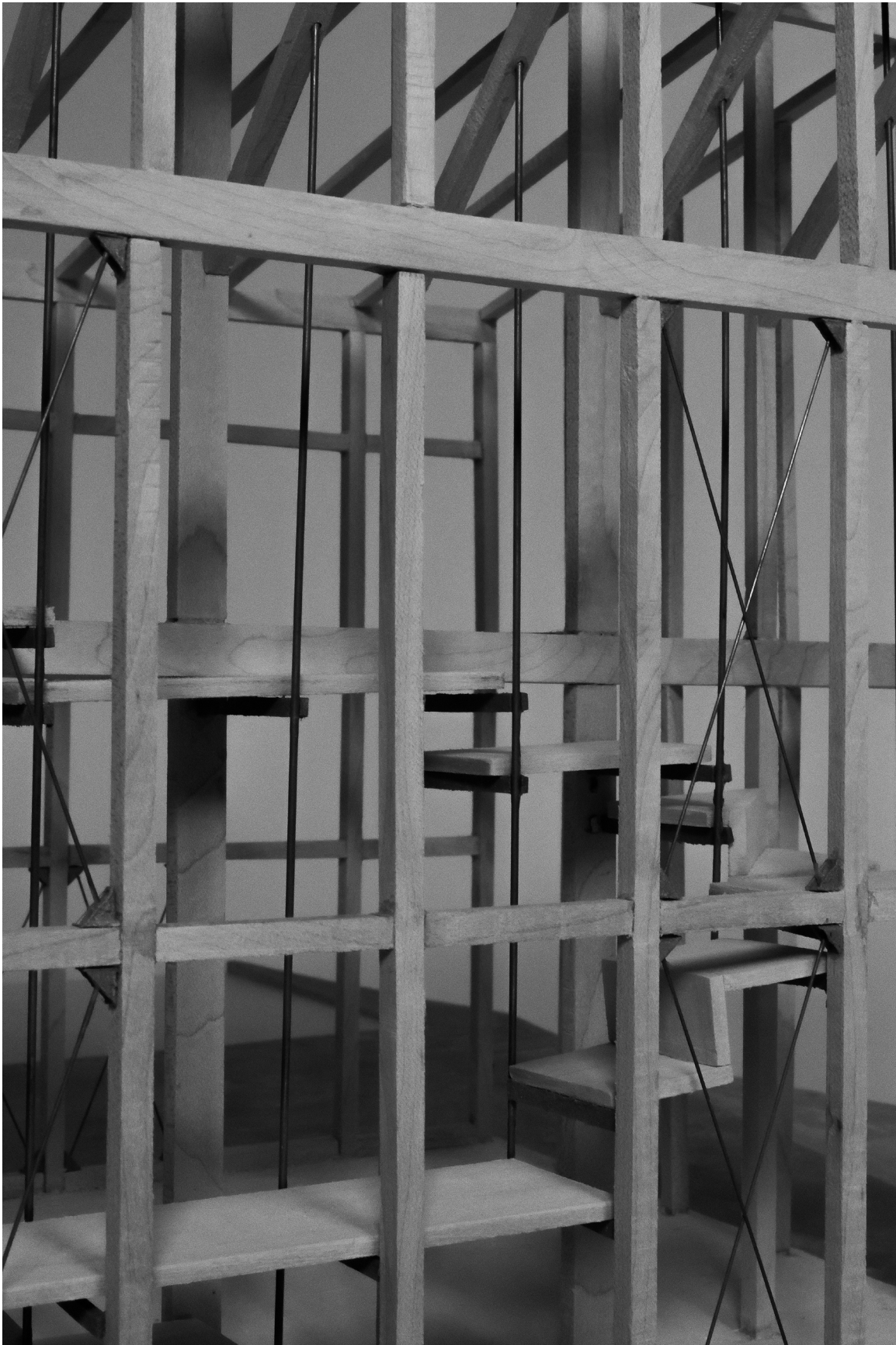
A close-up shot of the "stair hall" composed of wooden columns, beams, and girders with steel cable cross-bracing.
